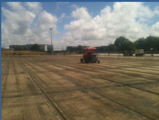
Slit drain installation at the Christchurch Temporary Stadium, Addington.
