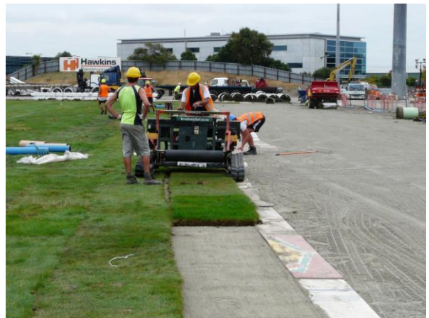
Relaying the AMI Stadium turf at the Christchurch Temporary Stadium, Addington.
